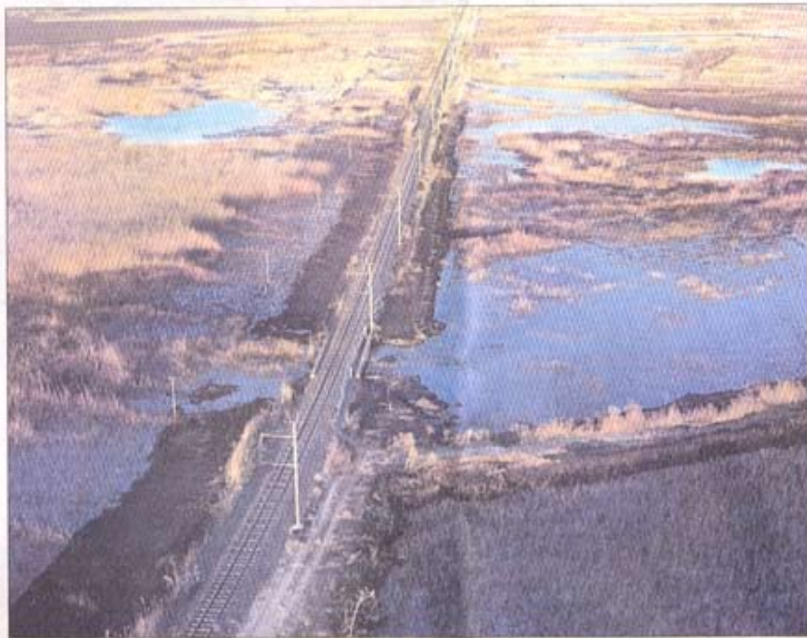
TROUBLE FOR TRAINS: While the process of upgrading the Homevale Sewerage Works has started, raw sewage is being pumped into the veld around Kamfers Dam, building up against the railway line, and flowing through a culvert into Kamfers Dam.
